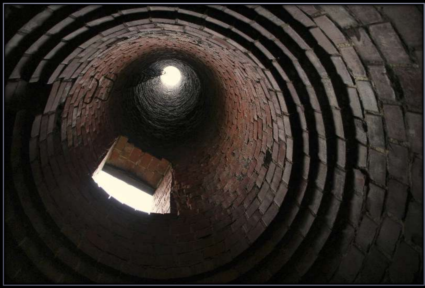
Abandoned United Distillers Chimney - Hebron, CT
