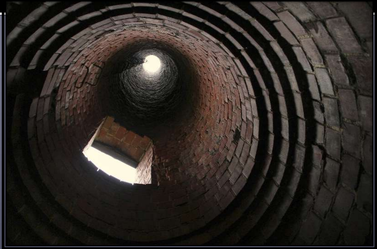
Abandoned United Distillers Chimney - Hebron, CT
