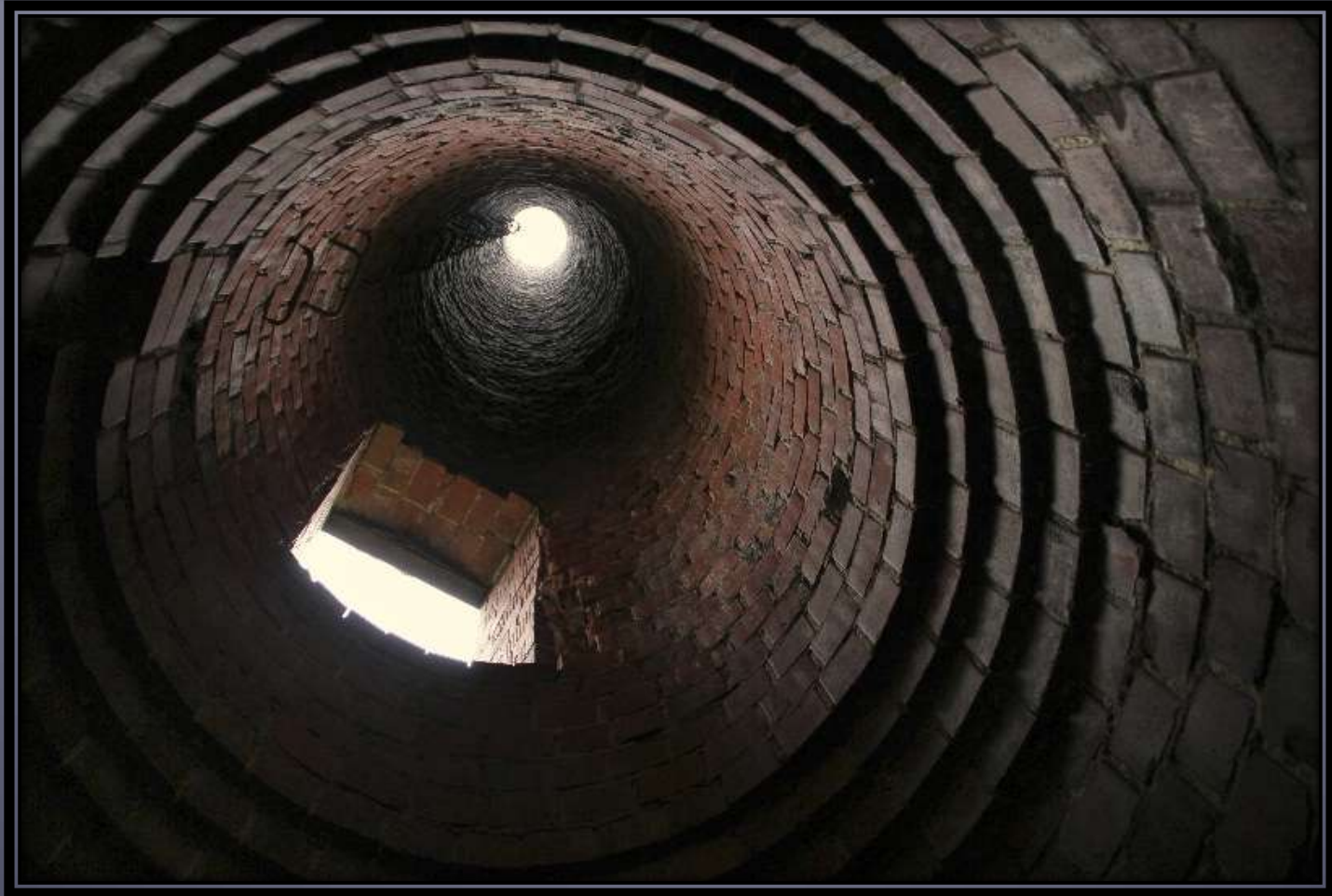
Abandoned United Distillers Chimney - Hebron, CT
